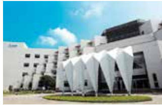
Tainan Plant (Diamond-rated Green Building)
